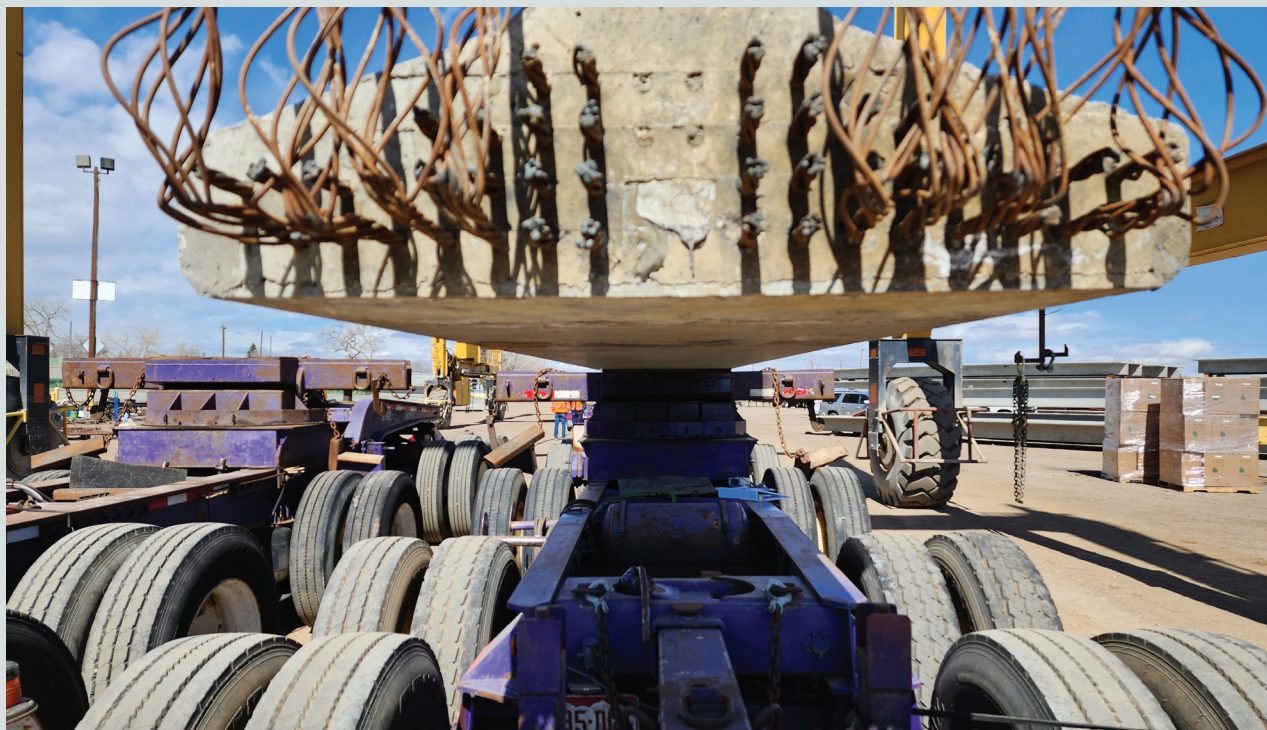
Figure 3. Girder placement on the vehicle.
